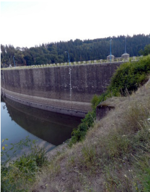
Photo 4. The dam on Pilchowice Lake. Photo by Zbigniew Piepiora.
