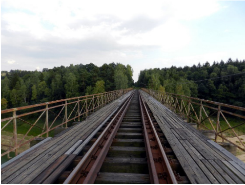
Photo 2. On the railway bridge over Pilchowice Lake. Photo by Zbigniew Piepiora.
