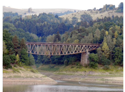
Photo 1. The railway bridge over Pilchowice Lake. Photo by Zbigniew Piepiora.
